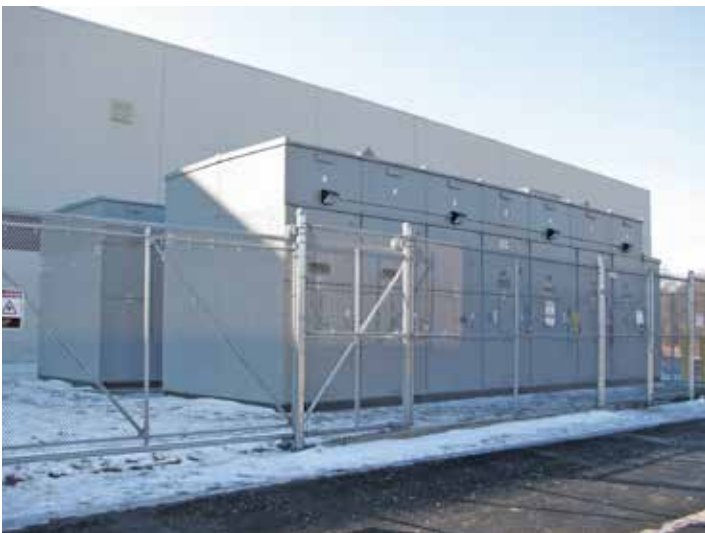
Metal-Enclosed 38 kV Switchgear 7-Bay Engineered Switchgear for Global Financial Leader
