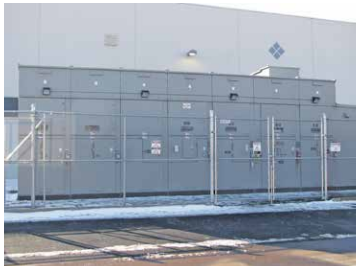
Metal-Enclosed 38 kV Switchgear 7-Bay Engineered Switchgear for Global Financial Leader
